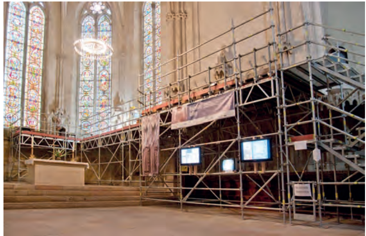
Fig. 7 Scaffolding installed for investigation in the west choir of Naumburg Cathedral. (Photo Dominik Jelschewski)
