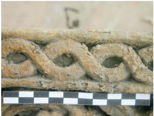
Fig. 5 Patan, Bhandarkhal Tank Pavilion, detachment of the surface and flaking due to a hydrophobic surface coating. (Institute of Conservation, University of Applied Arts Vienna, 2010)
